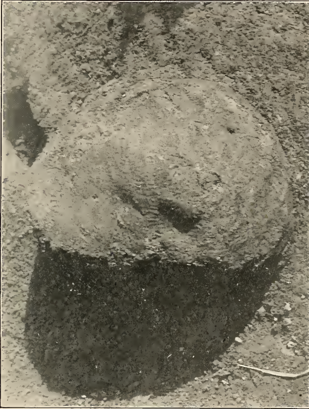
FIG. 116. AN INDIVIDUAL LOAD OF EARTH
